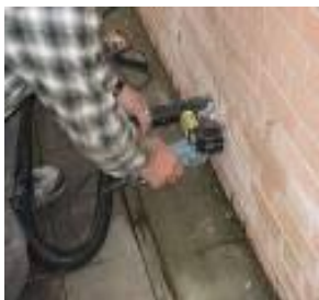
Tuck-point grinder With LEV
