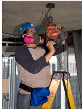
Drilling using a dust cap
