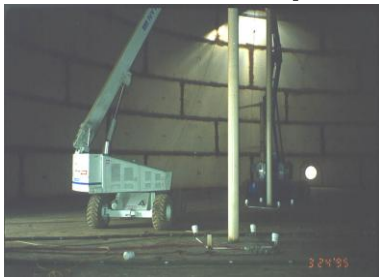
Propane powered Manlift in a large tank
