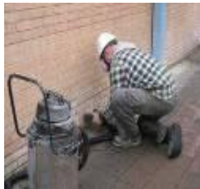
Tuck-point grinding With LEV
