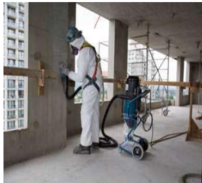
Wall grinding with LEV
