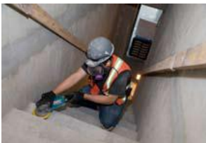
Stair grinding with LEV
