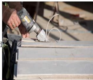
Cutting fiber-cement board with a hand-held shear
