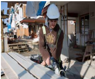
Worker cutting fiber-cement board outdoors, with a hand-held shear
