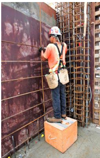
A simple platform, step, or ladder brings the work into a more comfortable, safer working height, optimally below shoulder height.
