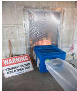
Poly enclosure with HEPA "negative air" unit
