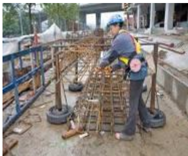
Prefabricate steel arrangements. This reduces forward bending.
