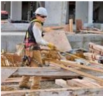
Raise materials to waist height. This reduces forward bending.
